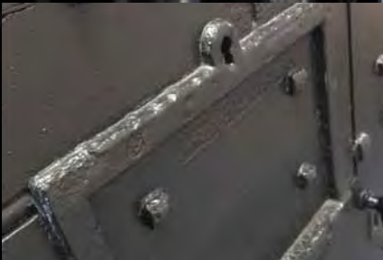
Lincoln Castle Prison cell door parts We used the existing ironmongery to make new patterns and produce castings for the gaol.
